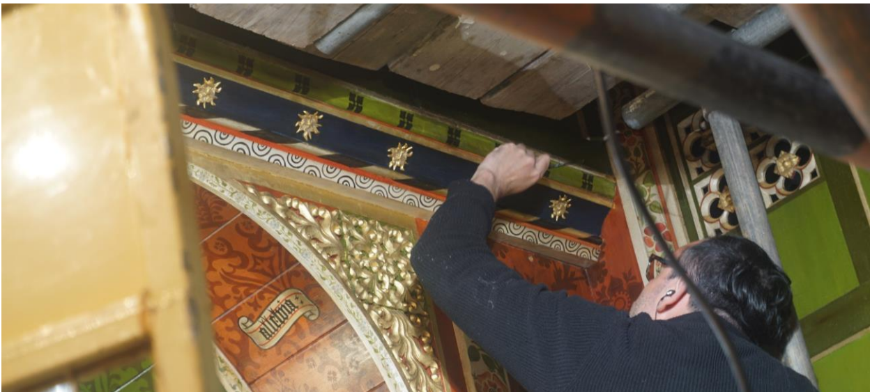
Details during application of the new stars and retouching of blue background.
