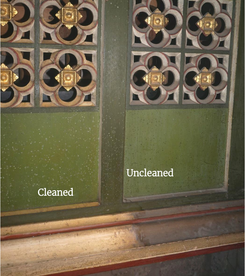
Details during cleaning of dirt and grime layers.
