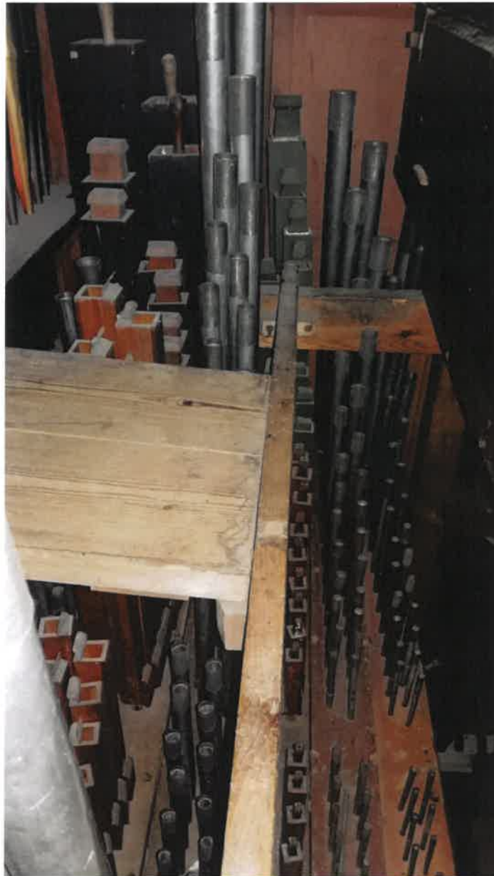
Great Organ pipework, with tuning platform and rear of façade pipes on the left and the Swell Organ expression box on the right
